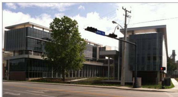
View of the CTRB from Gale Lemerand Drive.
